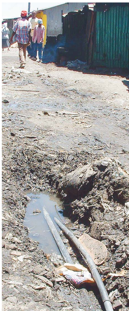
Pipes supplying water kiosks find their way through sludge and solid waste
